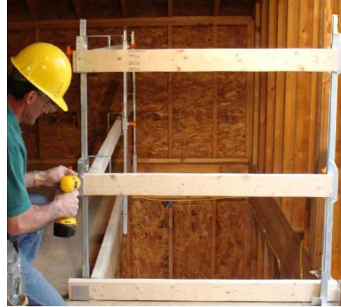
Figures 21 & 22 - Examples of guardrails installed around floor openings.
