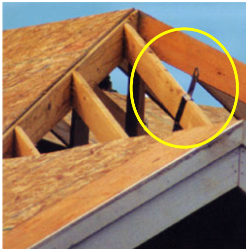
Figure 6 - A bolt-on anchor attached to a rafter.
