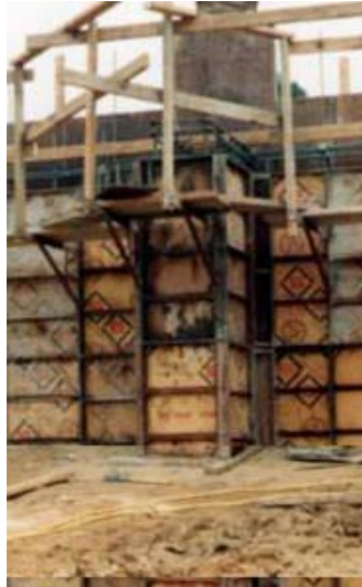
Figure 16 - A bracket-form scaffold attached to formwork.
