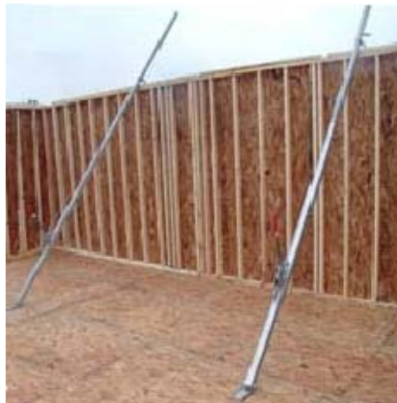
Figure 23 - Framed walls being erected using a jack.
