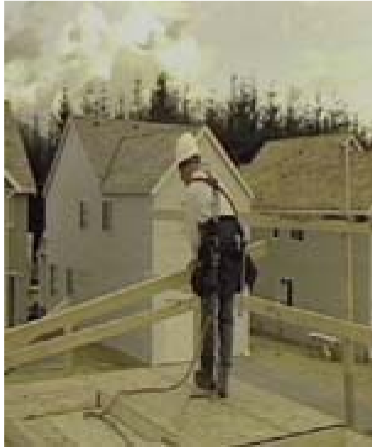
Figure 27 - Worker installing guardrails.
